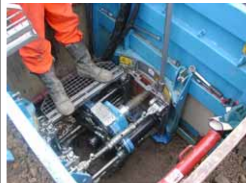
Installing the pilot bore.
