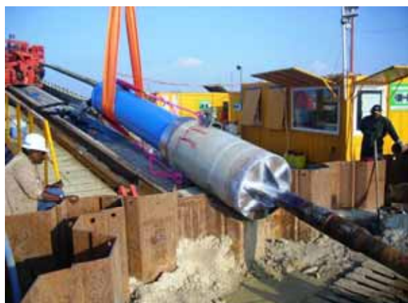
The TT-UK supplied Grundoram Taurus impact hammer set up on the end of the stuck drill string.
