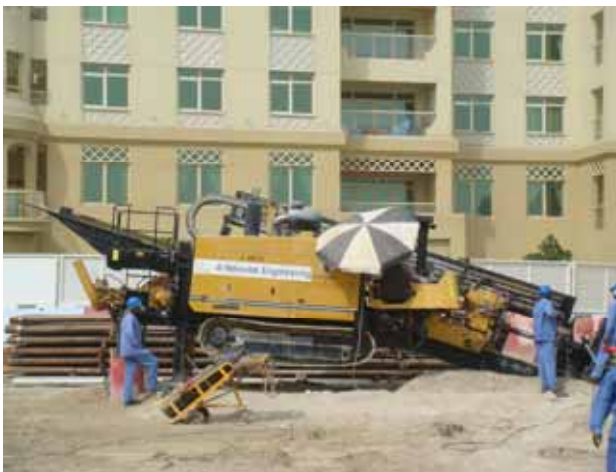
The Vermeer NAVIGATOR D100x120 drilling rig used for the smaller diameter boring work.
