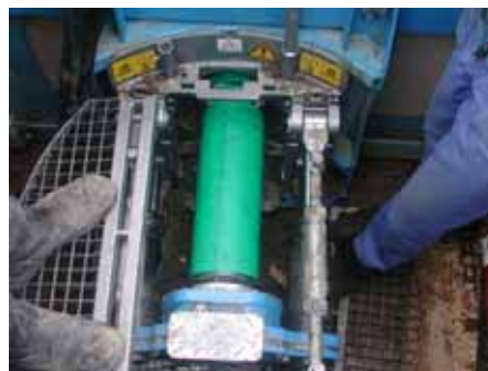
Installing the new pipe subsequent to the bore enlargement run.
