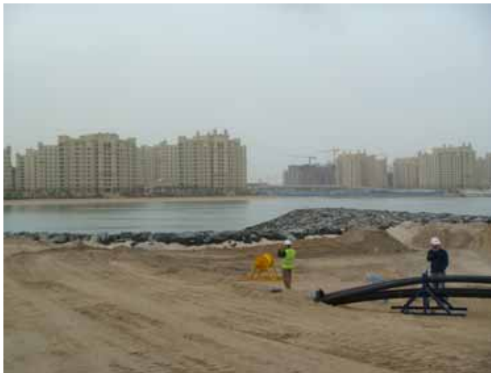
Pipe bundles are pulled into the casing pipes previous installed using HDD techniques.
