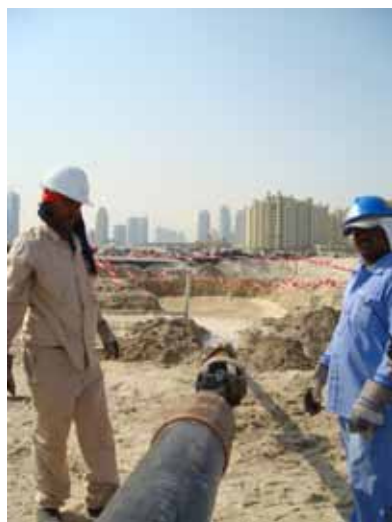
Ready to start the pipe pull-in with reamer head, swivel and pipe attached to the drill string.
